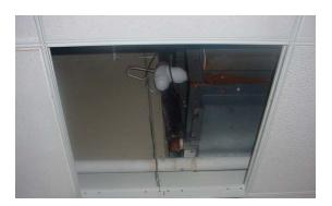
In the second incident, we observed a staff office where ceiling tiles had collapsed onto the desk of the staff member occupying the office. Fortunately, the staff member had stepped away from the office just before the collapse. The third incident also involved a collapsing ceiling tile. A ceiling tile in the office assigned to the OIG auditors appeared water damaged and ready to collapse. When lightly touched, the ceiling tile did in fact collapse.
