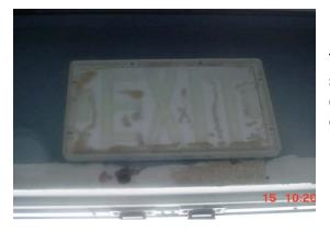
The picture on the left shows an inoperable exit sign in a dormitory. These exit signs are critical for escape in fire and other emergencies.
